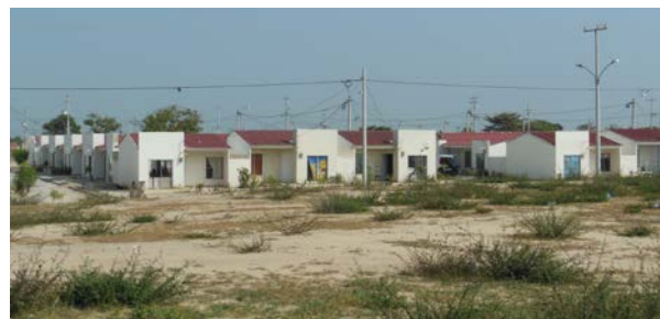
Picture 2. Nueva Esperanza housing project
