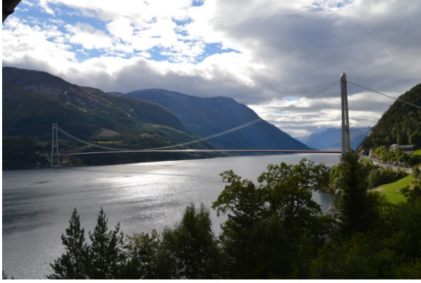
Fig. 3 The Hardanger Bridge
