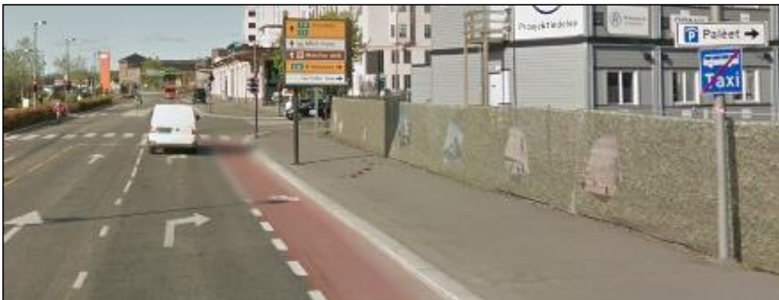
Figure 3: Termination of dedicated public transport lane at intersections in Norway. [Source: Google Maps – street view]
