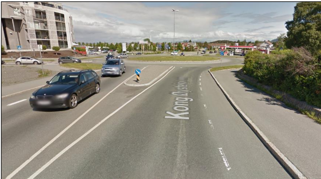
Figure 7: Termination of bike lane at a roundabout in Trondheim, Norway. [Source: Google Maps – street view]
