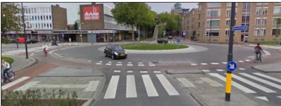
Figure 10: Priority of cyclists through a roundabout in the Netherlands. [Source: (State of the Art Bikeway Design – A further look, 2011)]
