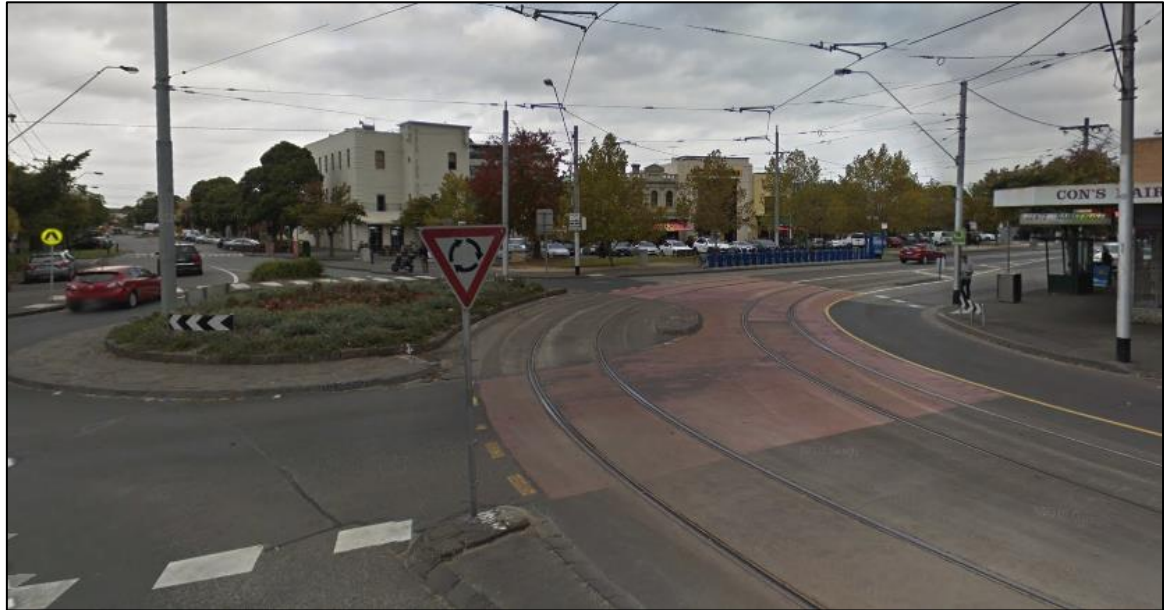
Figure 31: Coloured asphalt at conflict points in Melbourne, Australia. [Source: Google Maps – street view]
