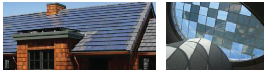
Figure 1. Examples of BIPV tiles (left) and BIPVs as solar cell glazing products for roofs (right) (Applied Solar 2010 [4], ASI® Glass photovoltaic modules Schott Solar AG [5]).
