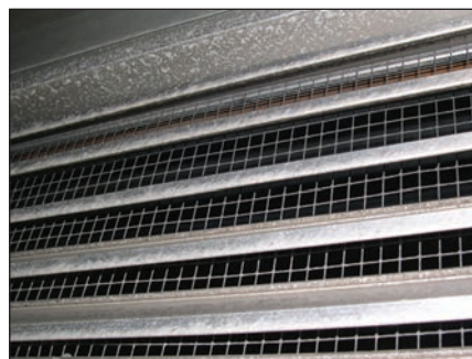
Photo 4: Closeup of metal grid and blinds from Photo 2 .
