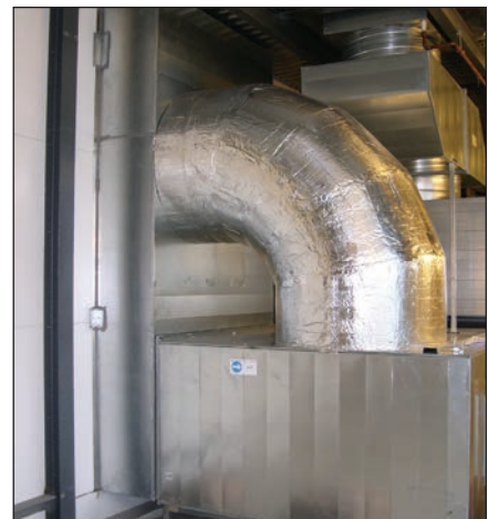
Photo 8: Inside the building at the intake (left) as shown in Photos 6 and 7 . The building was completed before the actual required air ventilation dimensions were calculated, resulting in too small dimensions for the ventilation system.
