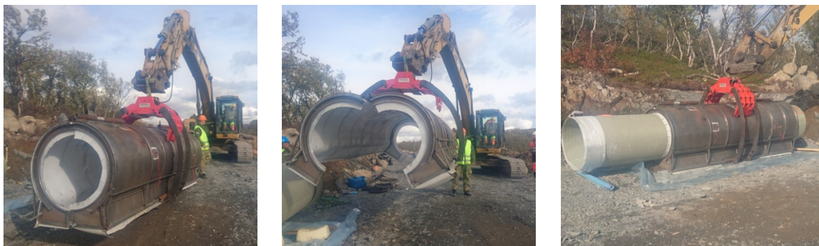
Figure 4: a) Closed "claw" b) The "claw" is opened c) Closed framework placed around the pipe
