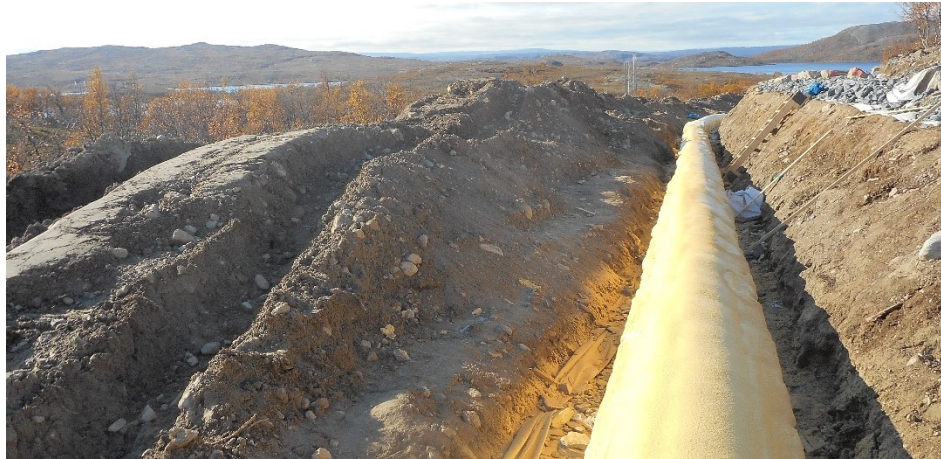
Figure 1 PU-foam used as backfill
