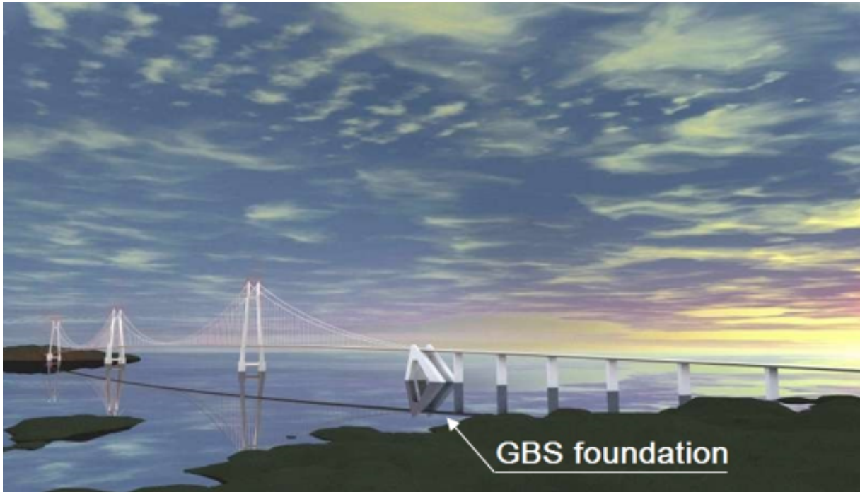
(a) GBS foundation of the bridge shown
