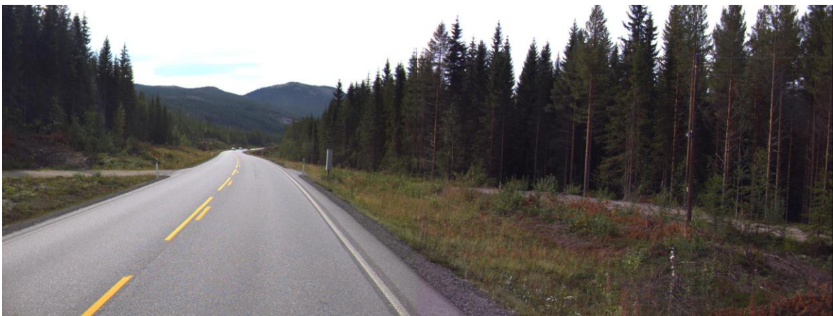
Figure 1: Image from one of the loop detectors
