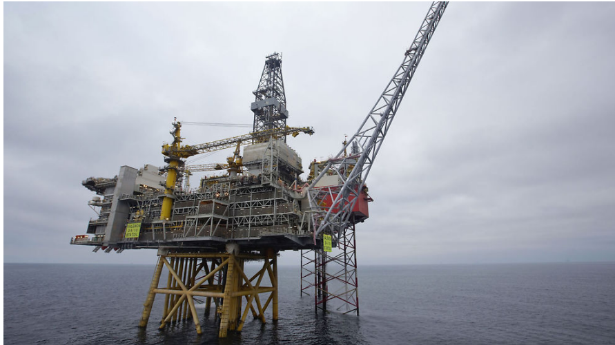
Figure 12: Valemon platform (Statoil, 2016b)
