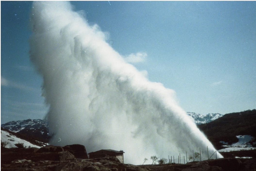
Figure 1-Outblow at Holmaliåna brook intake (Bekkeinntakskomiteen, 1986)
