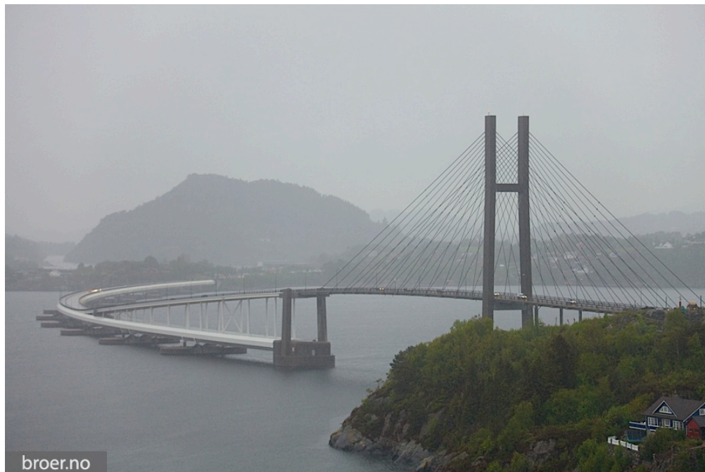
Figure 4: View of the Nordhordland bridge with the cable bridge, underpass and arced shape visible (Broer.no, nd)
