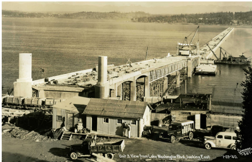
Figure 1: Construction of the Lacey V. Murrow Bridge (Washington State Archives, nd)
