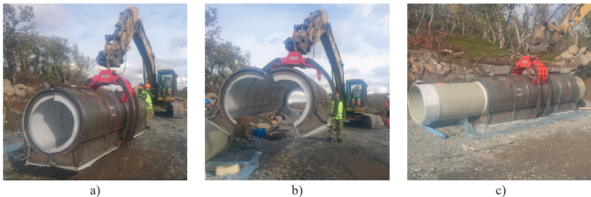
Figure 4: a) Closed "claw" b) The "claw" is opened c) Closed framework placed around the pipe
