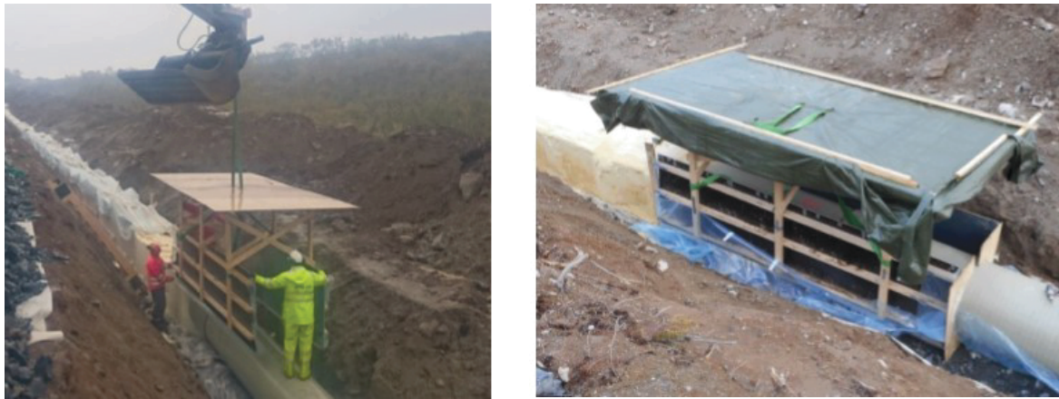
Figure 3: a) Formwork relocated with an excavator b) Formwork placed around the penstock
