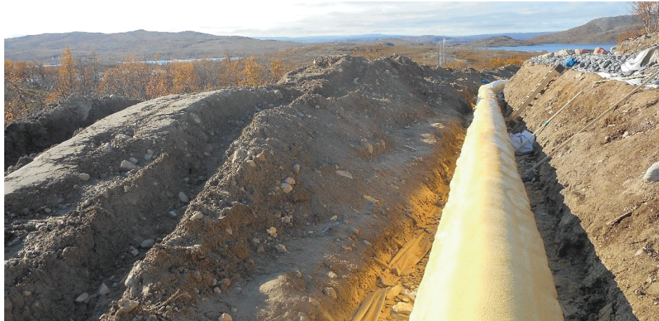
Figure 1 PU-foam used as backfill
