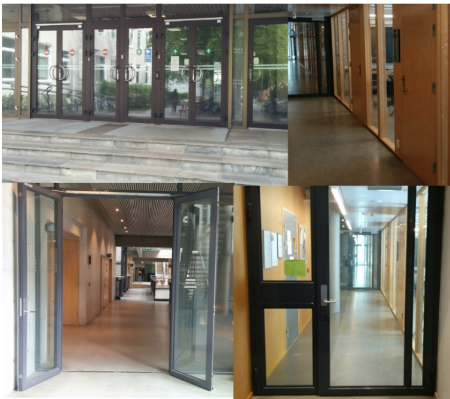
Figure 7.1: The different doors that the route passed through. Top right: Automatic doors, top left: door to the right of the path, bottom right: Open door, bottom left: Closed door.
