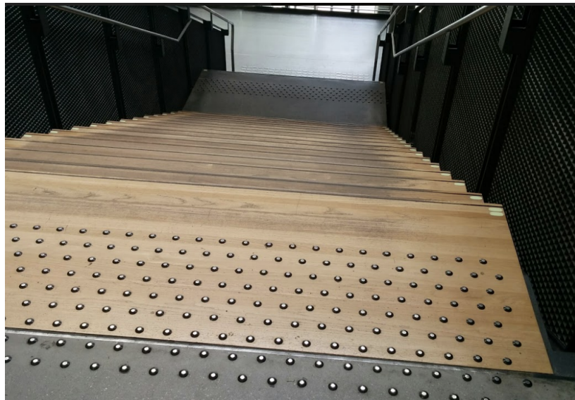
Figure 6.5: Tactile paving on top of the stairs used in the route.
