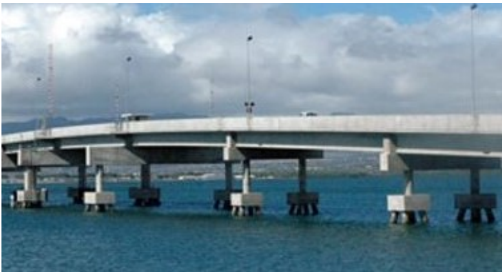
Figure 8: The Ford Island Bridge[15]
