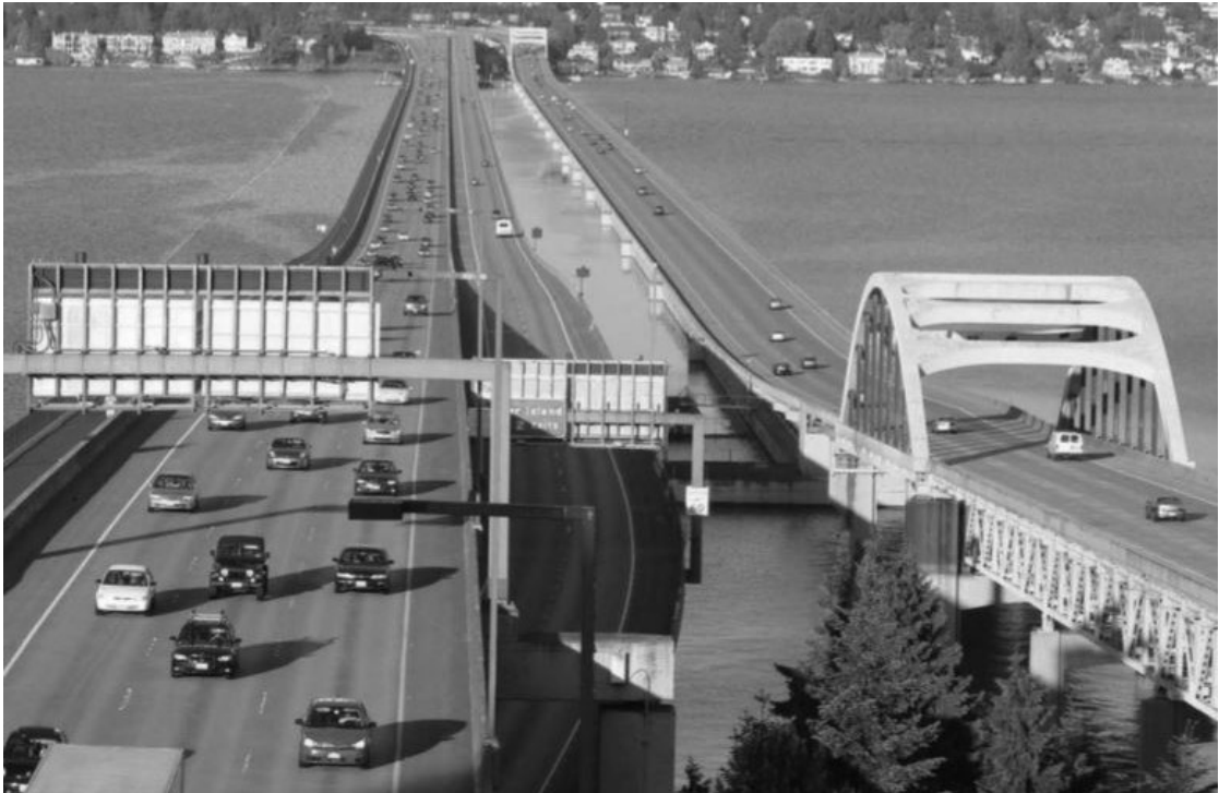
Figure 2: The Lacey V. Murrow Memorial Bridge at the right and the Homer M. Hadley Bridge at the left[7]
