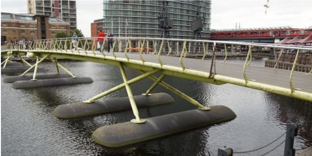
Figure 7: West India Quay Footbridge[14]
