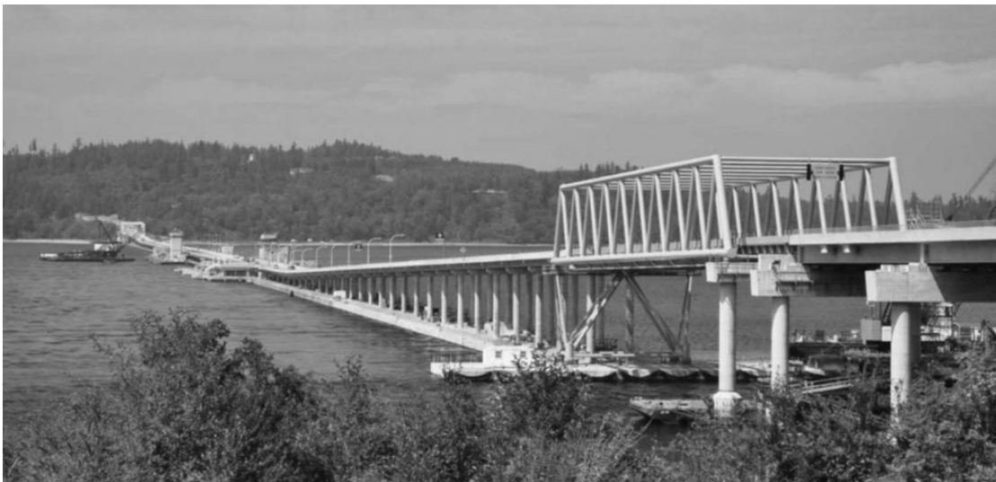
Figure 4: The new eastern half of the Hood Canal Bridge[7]
