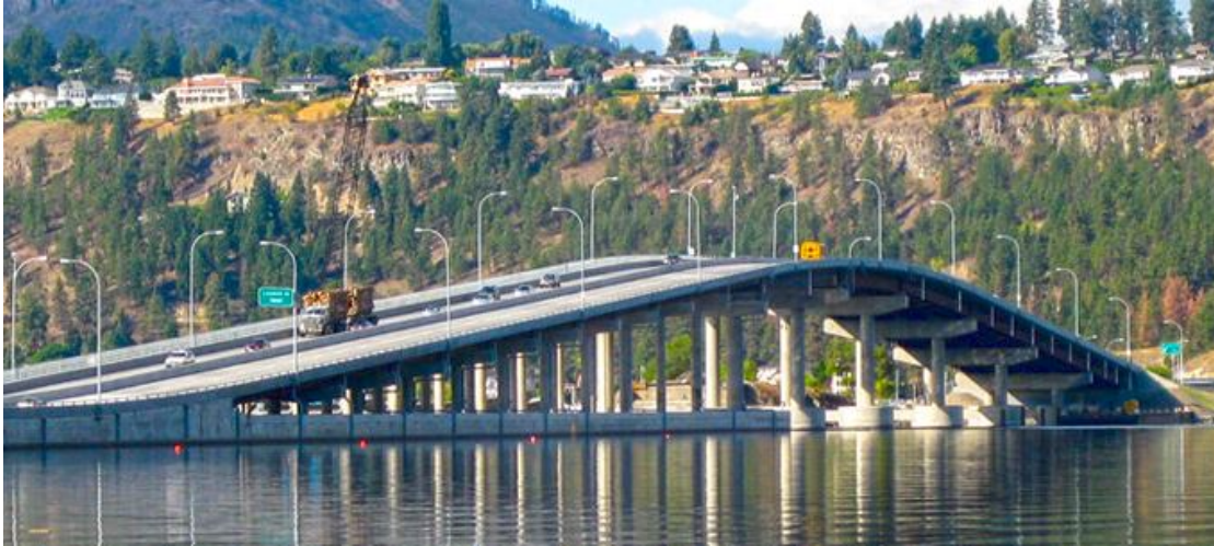
Figure 11: William R. Bennett Bridge[18]
