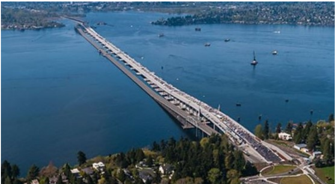
Figure 3: The Second Lake Washington Bridge[8]
