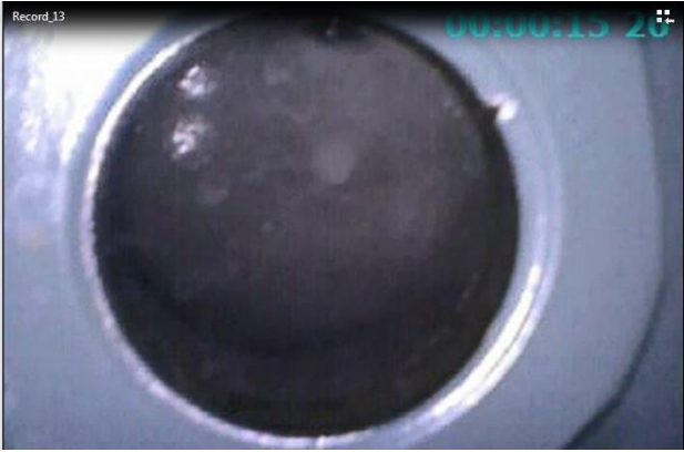
3. Superheat compressor suction 10K
