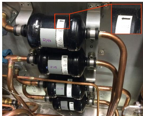
Figure 2.24: Filter driers for reversible R-744 heat pump
