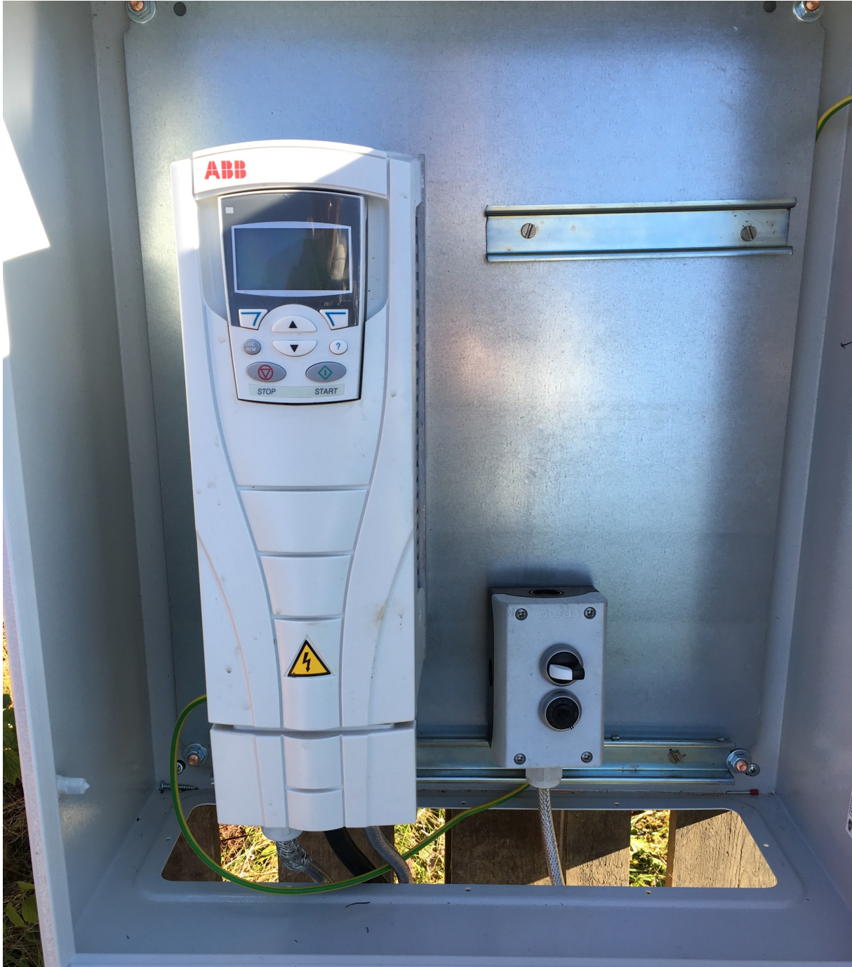
Figure B.9: Photograph of the frequency converter used for governing the motor and the potentiometer
