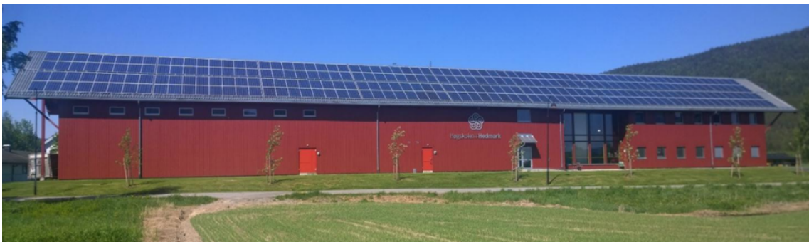
Figure 1.4: Picture of the PV system at Evenstad. Provided by Statsbygg.
