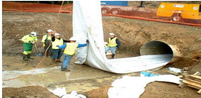
Figure 18: Deteriorated pipe being treated with cured-in-place lining (bing.com. cured-in-place lining)
