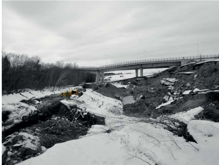
Figure 1-3 The quick-clay landslide caused by terrain work led to the collapse of the Skjeggstad bridge. The yellow bulldozer carrying out the work is seen in the left part of the slide pit. Photo: F. Oset
