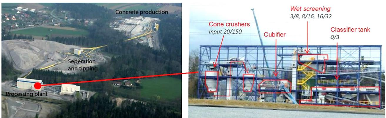
Figure 2-33: Left: Overview over Koralm KAT2. Showing the concrete production at tunnel portal. Secondly, separation and tipping of spoil (0/16 and 16/150). At last processing of spoil and storage. All connected by a conveyor system[22]. Right: The building of the processing plant and installing of the machinery.
