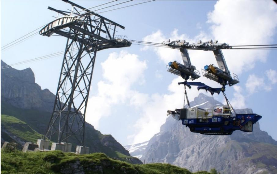
Figure 2-13: A 38 ton mobile impact crusher (swing-hammer) combined with a screening unit are being transported to the tunnel site (2500 ASL) at the Linthal-Limmern power station for the purpose of dry processing TBM spoil [61].
