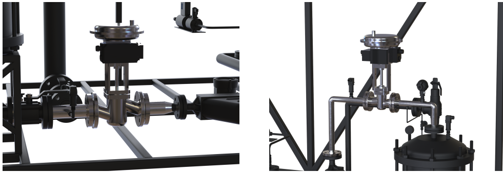
(a) 3-FV-201 control valve located at the joint water outlet.
