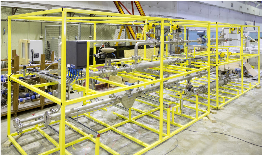
Figure 1.1: Phase 1 constructed facility [I].
