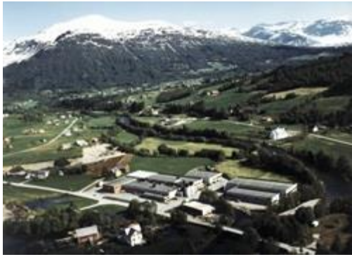
Figure 20 Grodås plant (Ekornes ASA, 2017)
