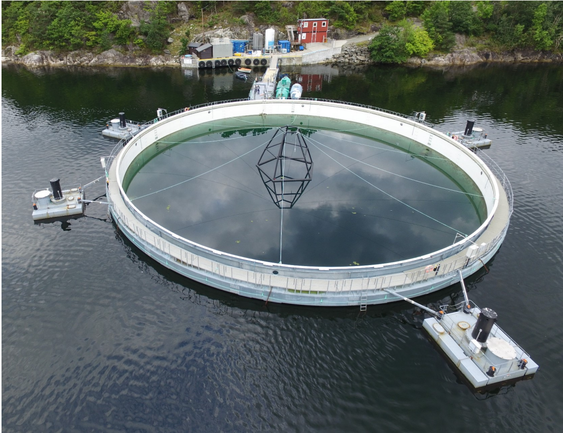
Figure 1.1: Neptun 3 closed fish farm plant located in Skaanevik, where Marine Harvest has its test production. The structure has a diameter = 40 meters and height = 22 meters (Kyst.no, 2016).
