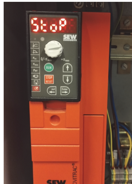
Figure 1-6 Frequency converter for fuel pump motor
