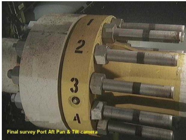
Figure 2.29: Bolted flange connector (Frazer et al., 2007).
