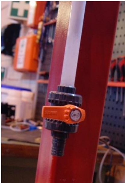
Fig. 3-21: The valve used at the bottom of the pipeline
