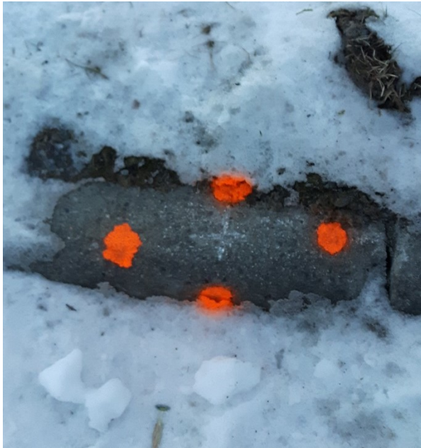
Figure 1.4 Kerbstone control point marking
