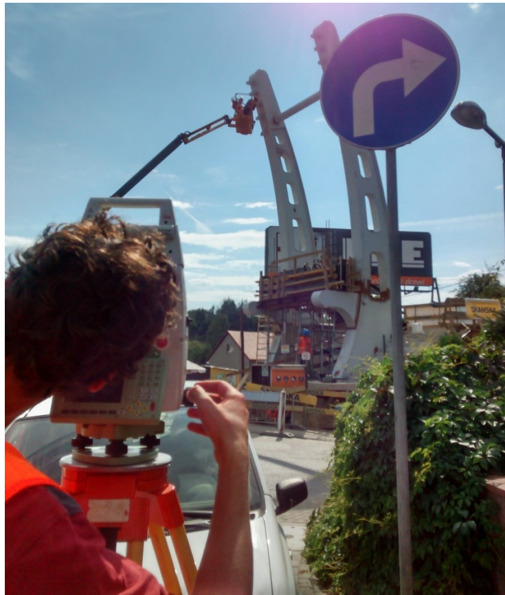
Figure 2.1 High precision, bridge hooks total station measurements
