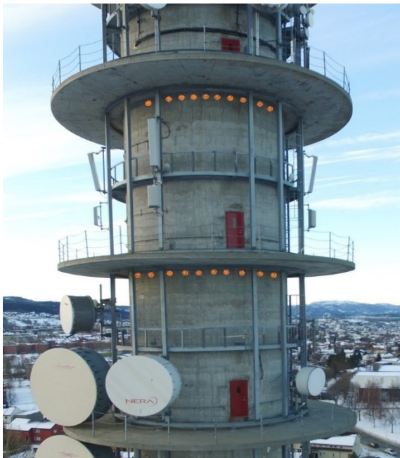
Figure 2.4 Total station cross-sections measurements placement
