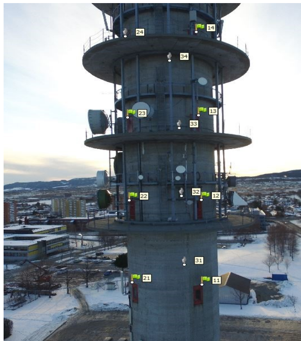
Figure 3.4 GCPs localization on a photo, Agisoft Photoscan
