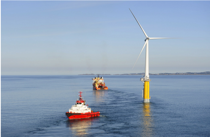
Figure 1.2.: HYWIND is towed into place. Photo: Øyvind Hagen, Statoil.
