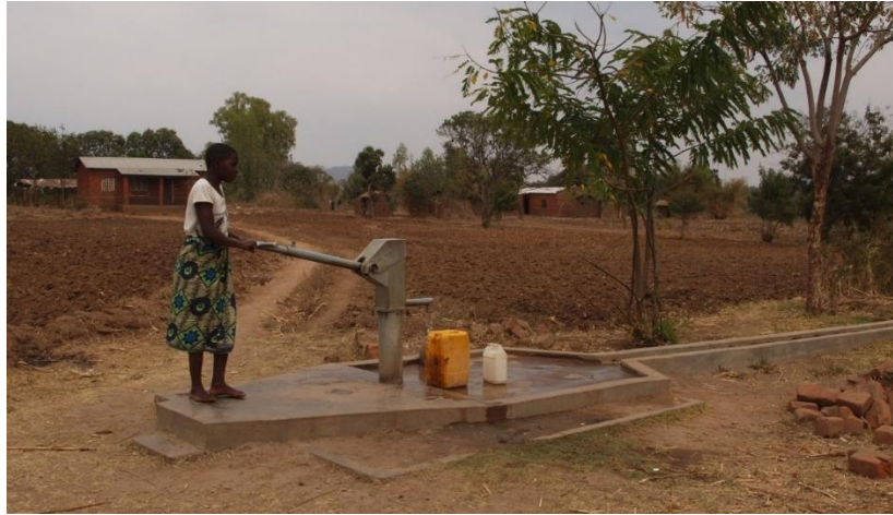
Figure 6.1: Photo showing the borehole in Mkhumba Village, Phalombe. This is the standard water pump found in both Phalombe and Nsanje (Photo: author).
