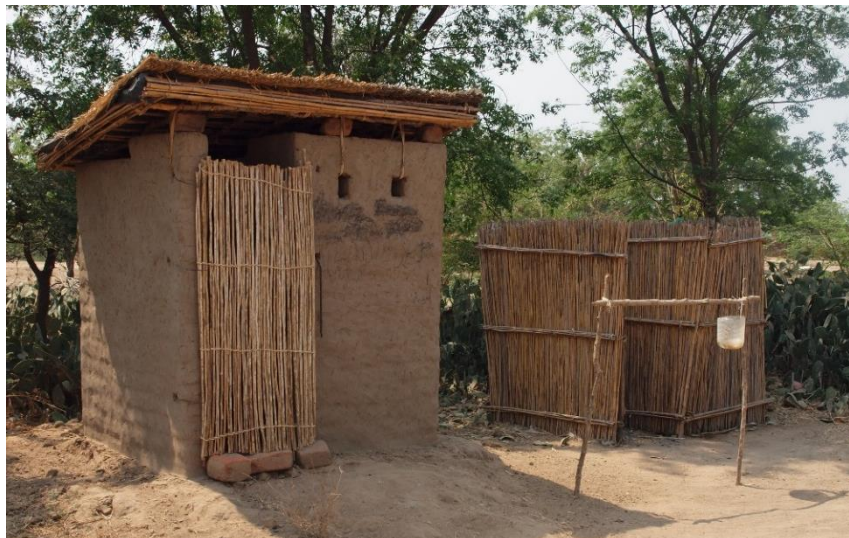
Figure 6.5: Photo of a reconstructed pit latrine with some washing equipment outside and a shower room – Alufandika Village, Nsanje (Photo: Author).
