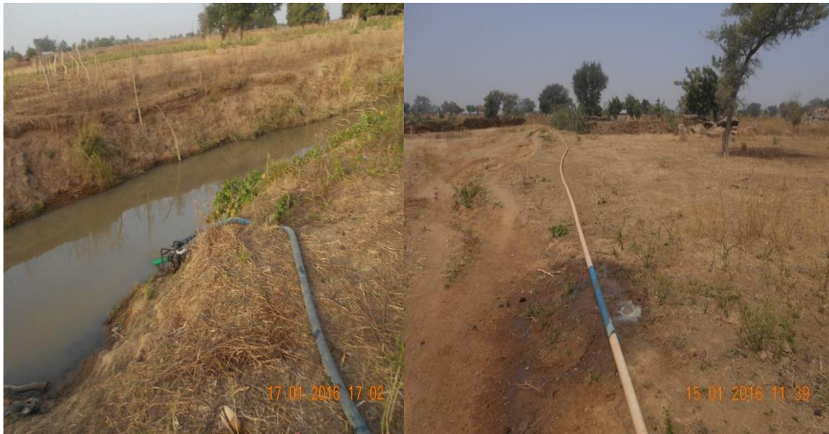
Figure 8: Photos of a pumping machine and pipes leading to farms
