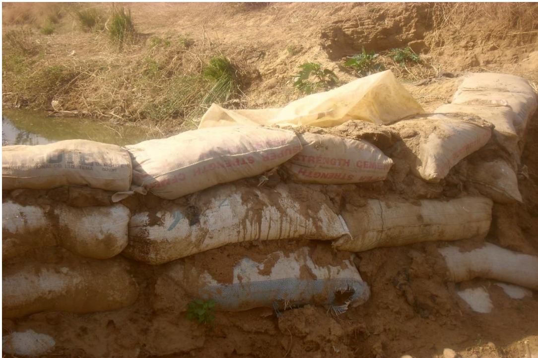
Figure 7: Photo showing water impoundment by farmers using bags of sand
