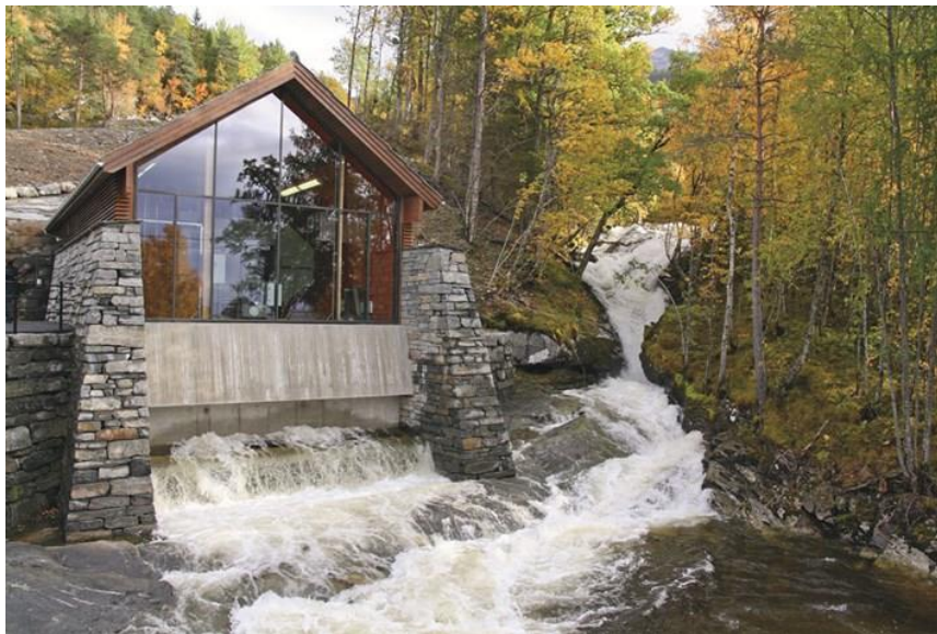
Figure 2.1 Ytre Alsåker power plant in Hordaland. Source: Statkraft (2015)
