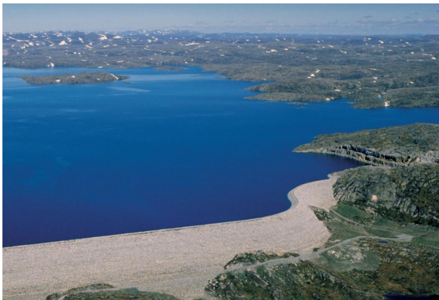
Figure 2.2 Blåsjø. Source: (Statkraft, 2013)
