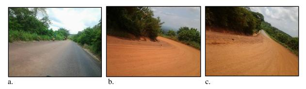
Plate 3 Meandering nature of the main road from Odumase<sup>49</sup> to the mine The photo on the left (a) shows a section of the road the slopes steeply and bends acutely as shown in the middle photo (b). The photo on the right (c) shows the continuous steepness of the road from photo b.
