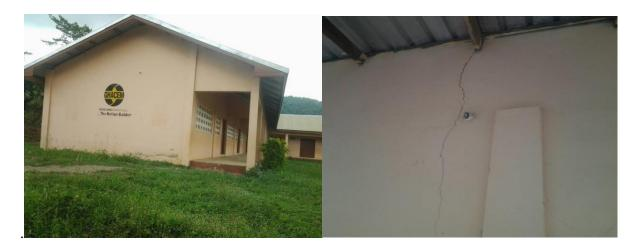
Plate 4 Cracked wall
