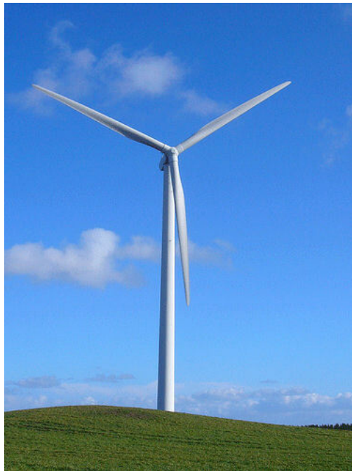
Figure 3.1: HAWT designed wind turbine.
