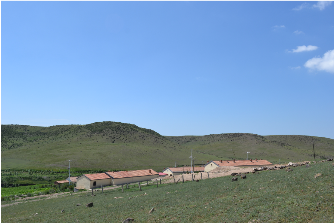
Picture 10 Houses of local people who live close to Han Wu La Wind Farm
