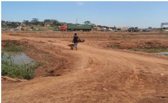
Figure 43: Road Construction in the wetland
