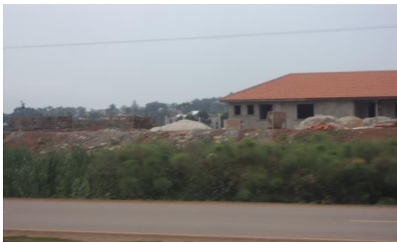
Figure 45: Sewage Treatment Plant in the swamp
