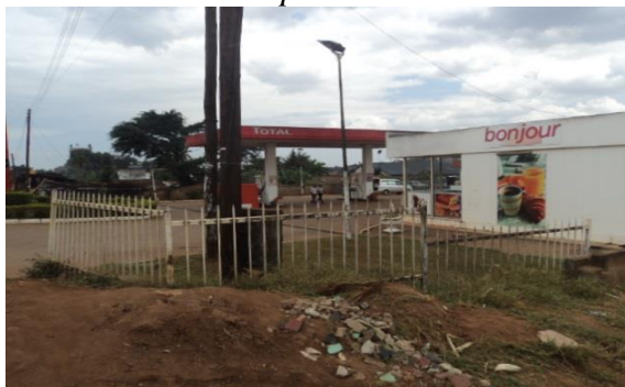
Figure 46: Fuel pump station located in low lying areas
