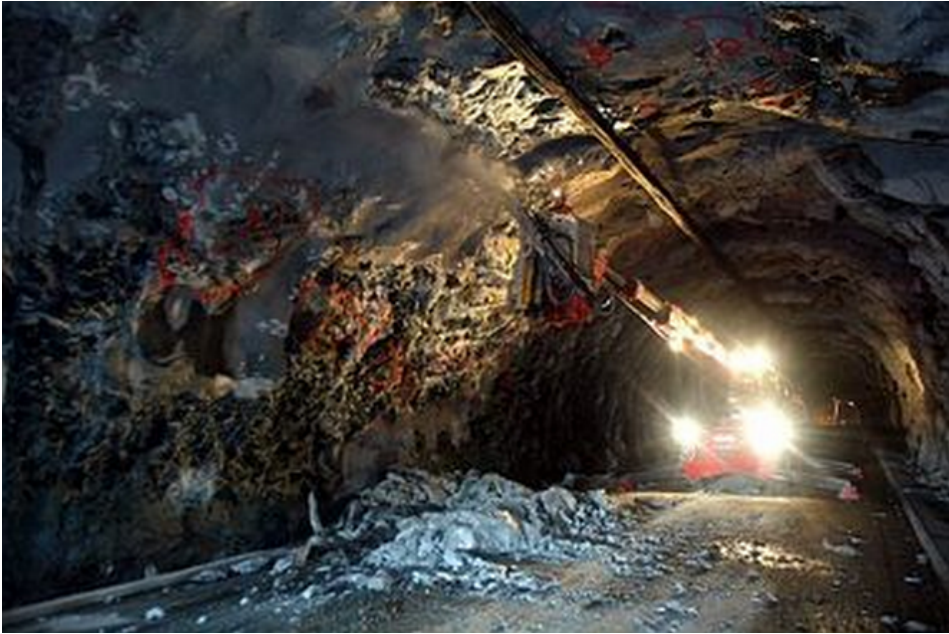
Figure 2.4: The Være-tunnel in Norway had stability issues both in constructional and operational phase due to difficult rock conditions. The picture is taken from the local newspaper after unstable rock mass had fallen on to the road (Adresseavisen[online], 2004).
