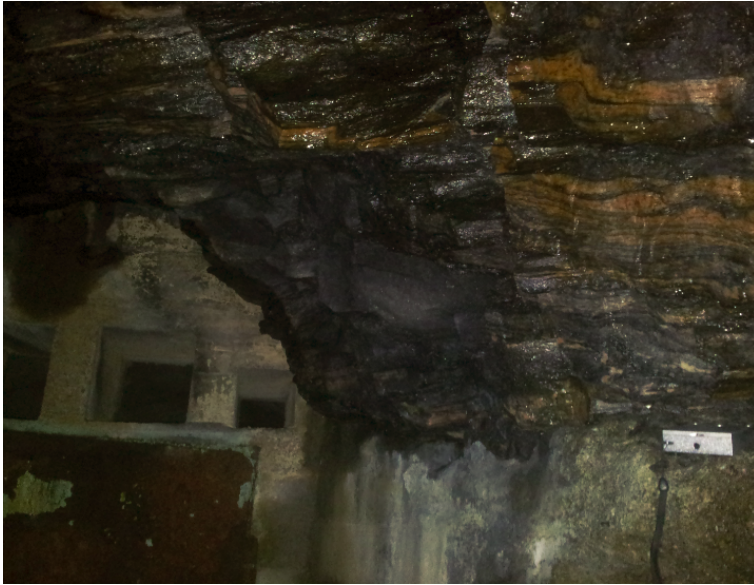
Figure 4.13: Image taken in the small tunnel in the mountainside just south of the city centre. Picture shows wet rock surface. It had not rained in the area in 4-5 days.
