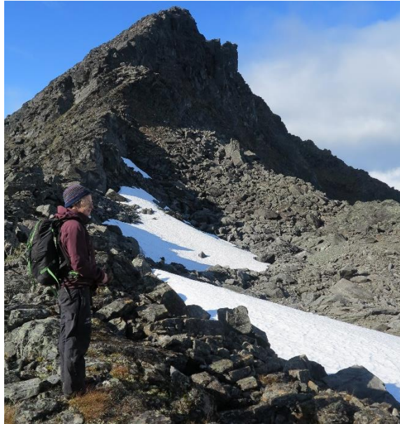
Figure 5.1 View towards west along the back scarp of scenario 3.A. Note the drop along the back scarp, and that the material that has dropped down is sloping towards the back scarp.
