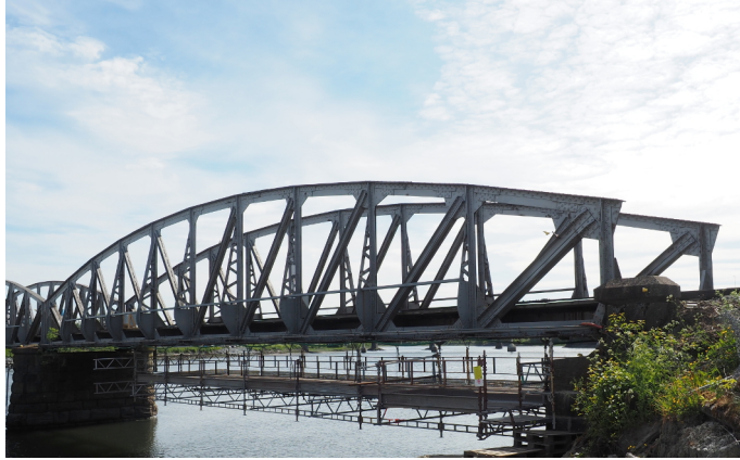
Figure 5: Hell railway bridge.
