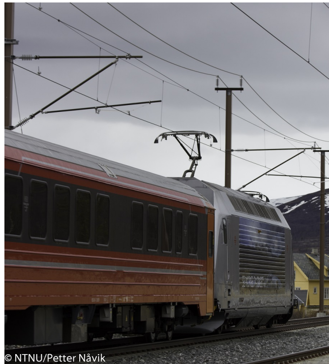
Figure 1: The catenary system, and the train [8]
