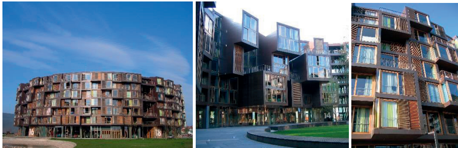
Figures 9(a), 9(b) and 9(c). Similarities in scale, proportion, materialization, rhythm and facade roughness. Student housing, Copenhagen, Denmark. Figures: Fernanda Acre.
