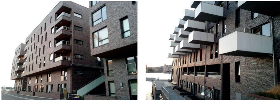
Figures 18(a) and 18(b). Balconies placed on top of each other (18a) and staggered balconies (18b). Residential building, Oslo, Norway. Figures: Fernanda Acre.
