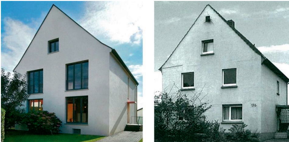
Figures 28(a) and 28(b). Changes in windows' size, after (28a) and before (28b) the dwelling renovation. Private dwelling, Bochum, Germany, © [Jörg Hempel]. Reproduced by permission of Jörg Hempel.
