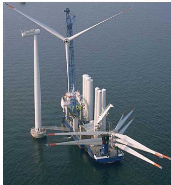
Figure 1.1: Offshore Windmill Construction
