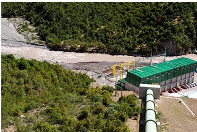
Figure 2.12 La Higuera Hydropower Plant (Statkraft)
