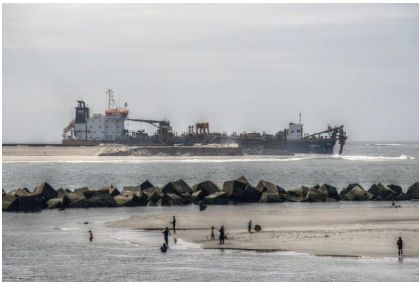
Figure 4.4 From the construction of Maasvlakte 2 (source: Wikipedia)
