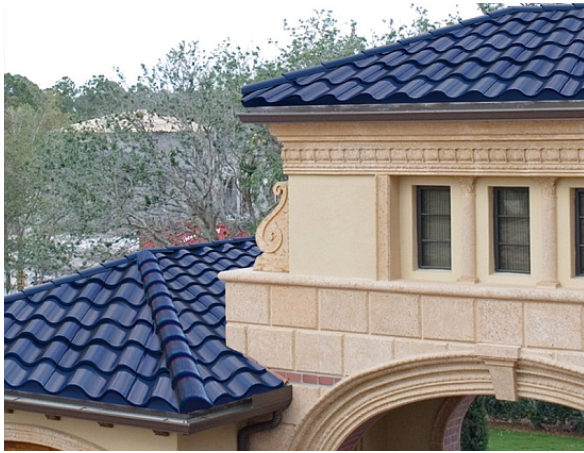
Figure 3: Curved clay looking solar tiles (Solar Thermal Magazine 2010).
