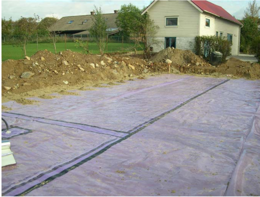
Fig.1. Placement of radon barrier under thermal insulation under baseplate of building.
