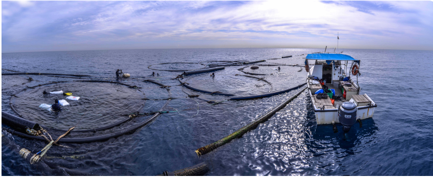
Figure 1.6: Collapsed fish farms due to harsh weather. ( www.thetower.org )
