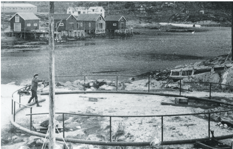
Figure 1.1: Manufacturing of the floater of the first Polarcirkel cage in 1974. (AK-VA group)
