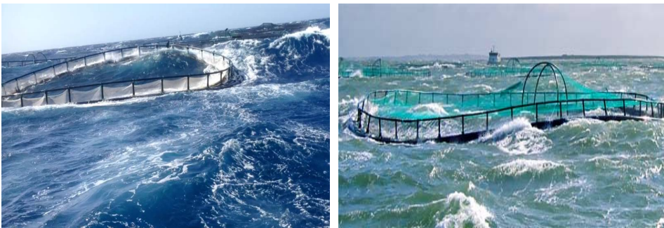
Figure 1.8: Open cage fish farm of circular floating collar of HDPE in bad weather. Large elastic deformations of the floater are clearly seen. (Left: Fusion Marine; right: Hvalpsund Net AS)
