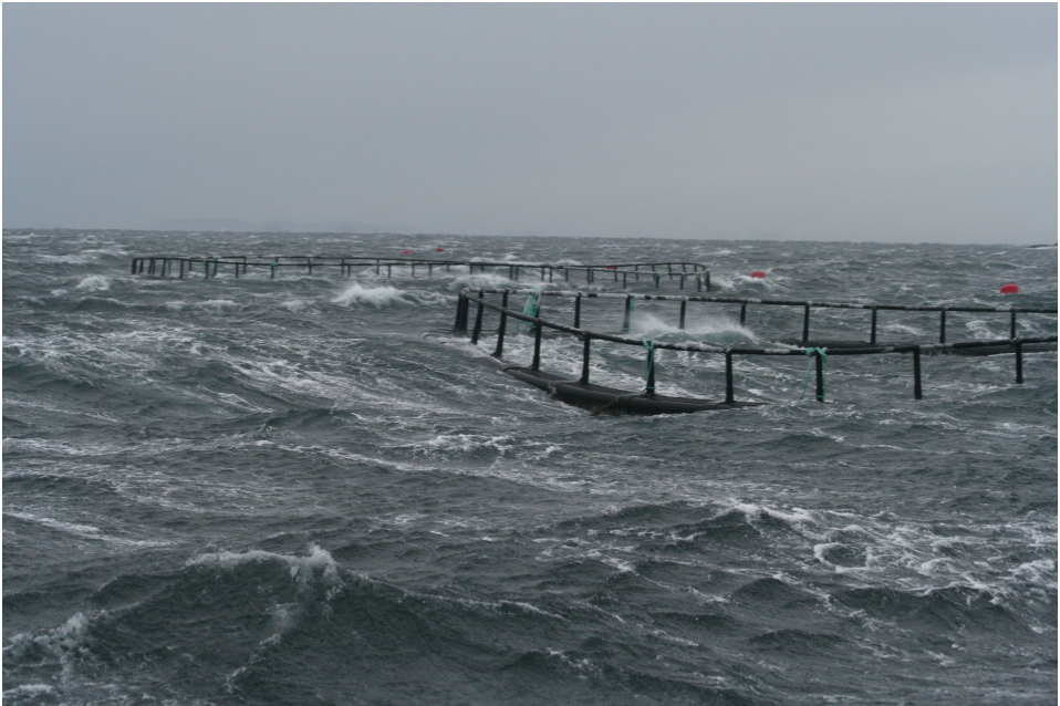
Figure 4.11: Illustrations of overtopping and out of water on the torus of a fish cage without net in a storm. (Photo: Marius Dahle Olsen)
