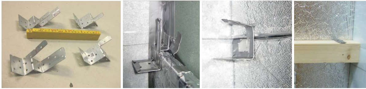
Figure 5. Principle of the fastening bracket. The left photo shows the fastening brackets used in the middle of the wall (between two VIPs, fastened on a wooden stud), and fastening brackets used at the top plate. The three other photos show different stages in the installation of the fastening bracket between two VIPs.
