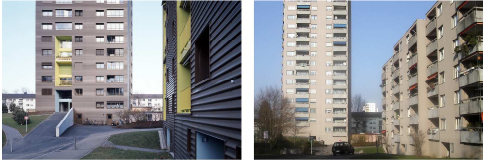
Figures 15(a) and 15(b). Changes in materialization of facades and windows' size and composition. Residential blocks, Zürich, Switzerland. Residential block after renovation (15a) © [Andrea Helbling, Arazebra]. Reproduced by permission of Andrea Helbling, Arazebra, Zürich. Residential block before renovation (15b) © [Schneider Studer Primas GmbH]. Reproduced by permission of Schneider Studer Primas GmbH.
