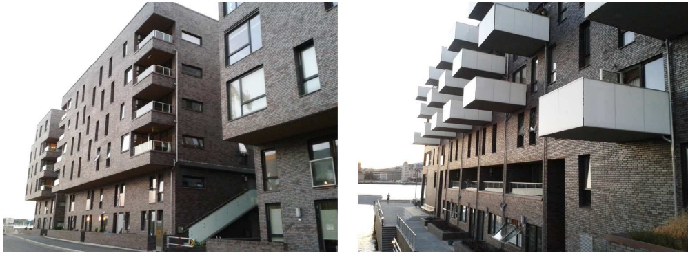
Figures 5(a) and 5(b). Balconies placed on top of each other (5a) and staggered balconies (5b). Residential building, Oslo, Norway, picture: Author. 178x65mm (300 x 300 DPI)
