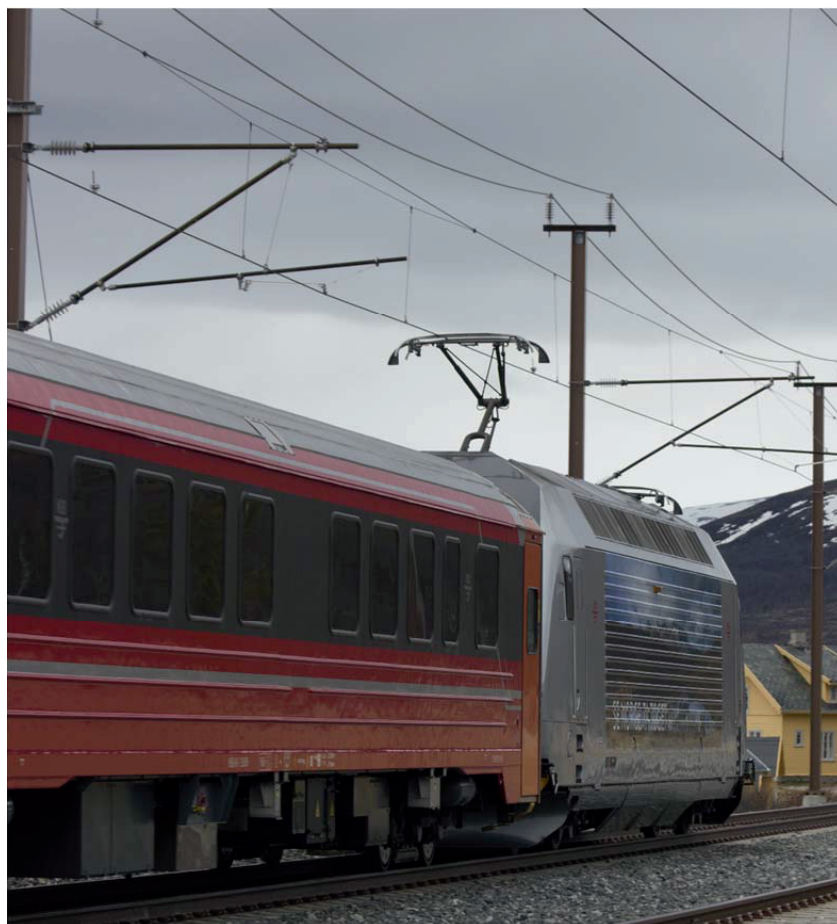
Figure 4. A train passing a catenary section. Photograph: NTNU/Petter N avik
