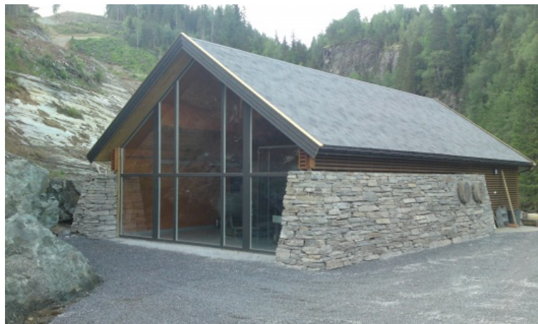
Figure 5.5: Bruvolllelva Power Plant
